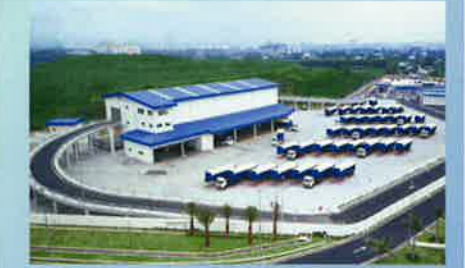
Kuala Lumpur Refuse Transfer Station (Malaysia)
