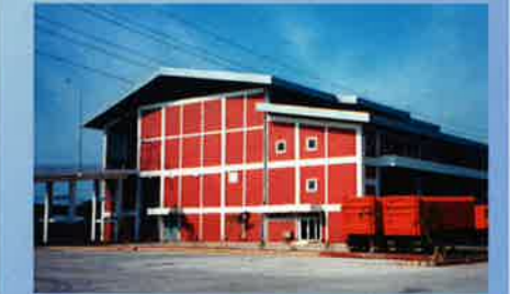
Jakarta Refuse Transfer Station (Indonesia)
