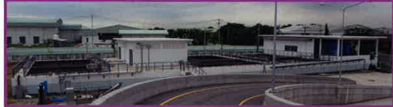
Water Treatment Building
