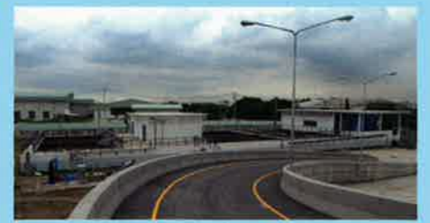
Water Treatment Building
