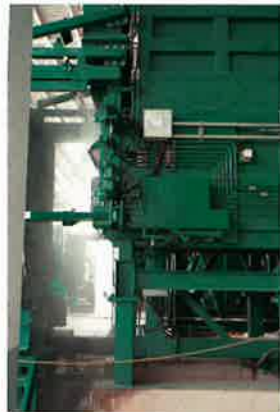
Compactor (Front portion)
