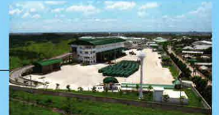
Bangkok Refuse Transfer Station
