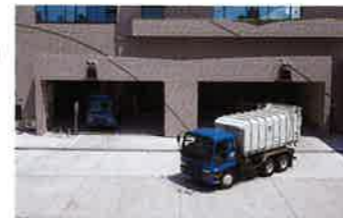
Shinjuku Refuse Transfer Station, Tokyo
