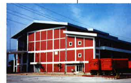
Jakarta Refuse Transfer Station
