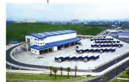
Kuala Lumpur Refuse Transfer Station
