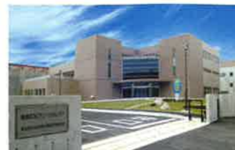
Nanbu Regional Clean Center, Takamatsu
