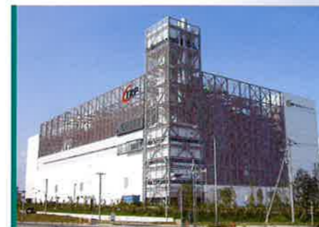
The Vertical Incinerator has been adopted for Super eco-town plant in Tokyo.
