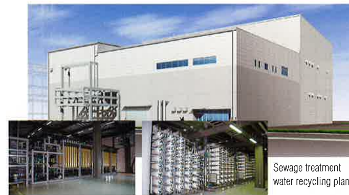
MF Membrane Unit RO Membrane Unit Wastewater recycling system with membrane technology. Sewage treatment water filtrated with membrane can be reused as industrial water.
