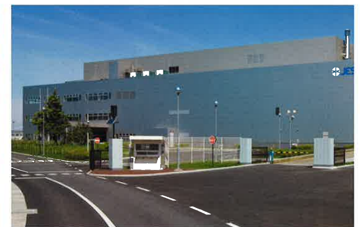
Japan Environmental Safety Corporation Hokkaido PCB Waste Treatment Facility
