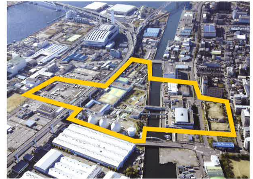
Sewage treatment plant (photo provided by the Kobe City Construction Bureau)
