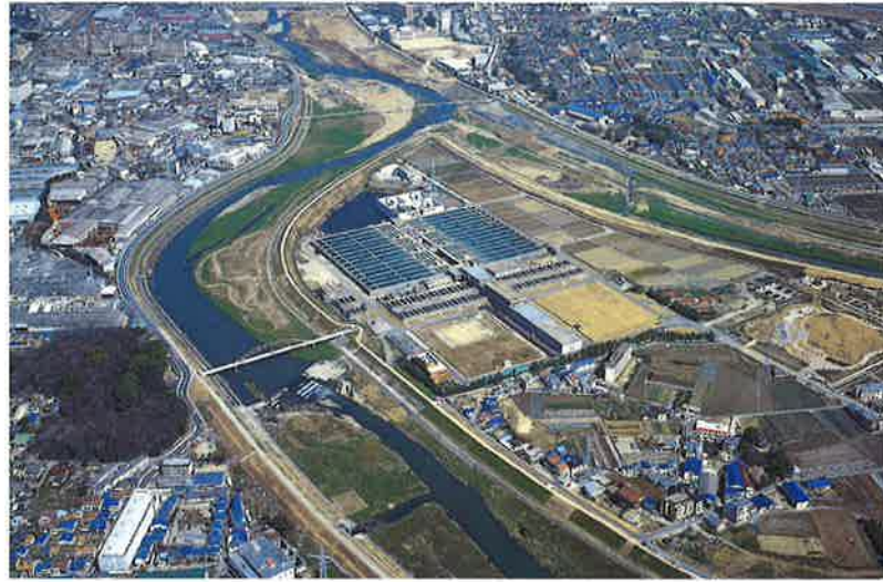
Water purification plant
