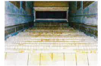
Inside the furnace
