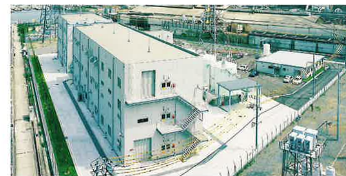
The Chugoku Electric Power Co., Inc Insulating Oil Recycling Center
