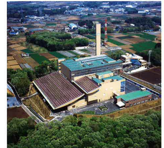
Tobu Clean Center, Tokorozawa city 115 tons/day × 2 furnaces (JFE Hyper Grate), 2,500kW of power generation, completed in 2003.
