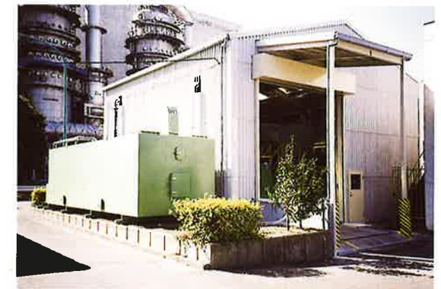
Hodogaya, Advanced Compost Production System, Yokohama completed in 1994
