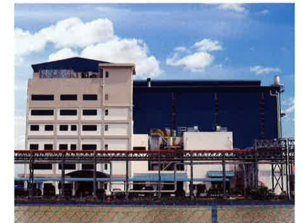
Genting Sanyen Industrial Paper SDN BHD , The model project for waste treatment of paper sludge and utilization of waste heat from combustion of paper sludge in Malaysia. 237.7 tons/day × 1 furnace, 17.3 tons/h saturated steam generation at 2.25MPa, completed in 2003.
