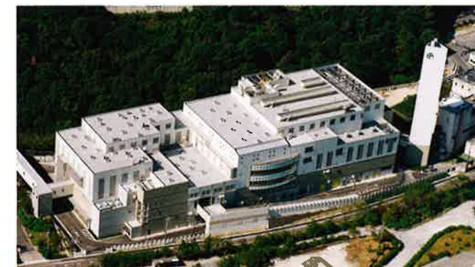
Kasugai Clean Center, Kasugai city 140 tons/day × 2 furnaces (JFE Hyper Grate), 7,000kW of power generation, with 40 tons/day Ash Melting Furnace (bottom ash and fly ash), completed in 2002.
