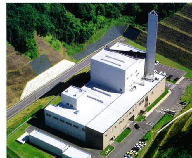
Hidaka chubu environment center, Hidaka chubu sanitary union. 20 tons/day × 2 furnaces (JFE High-Temperature Gasifying and Direct Melting Furnace) . With a heat recovery system for the air conditioning of the facility, completed in 2003.
