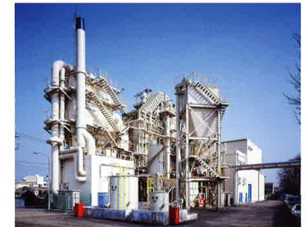
Hamura Clean Center 60 tons/day × 1 furnace, for general industrial waste, plastics and paint, and sludge, etc., completed in 1992.
