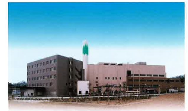
Hachioji Tobu Refuse Disposal Center. Metro. Tokyo 100 tons/day × 3 furnaces (JFE Hyper Grate), 1,990kW of power generation, with 36 tons/day Ash Melting Furnace (bottom ash), completed in 1998.
