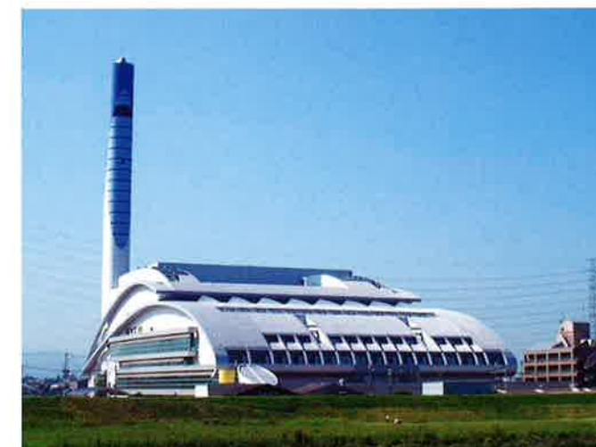
Hirano Incineration Plant, Osaka city 450 tons/day × 2 furnaces (JFE Hyper Grate), 27,400kW of power generation, completed in 2003.
