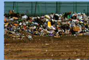
Excavating waste from final disposal site
