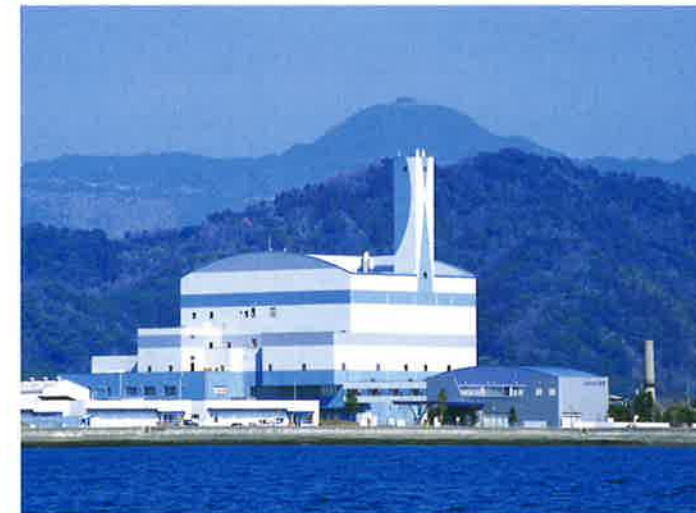
ECO CENTER BANJYO, Saiki area kouiki waste administration union 55 tons/day × 3 furnaces (JFE High-Temperature Gasifying and Direct Melting Furnace) . 1,600kW of power generation, completed in 2003.
