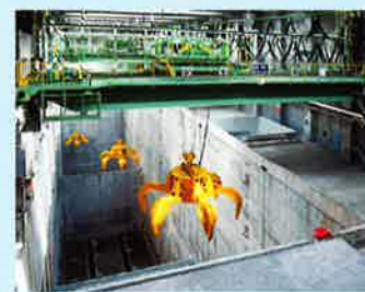
C Waste pit/waste hopper
