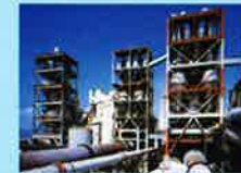
Raw materials for cement
