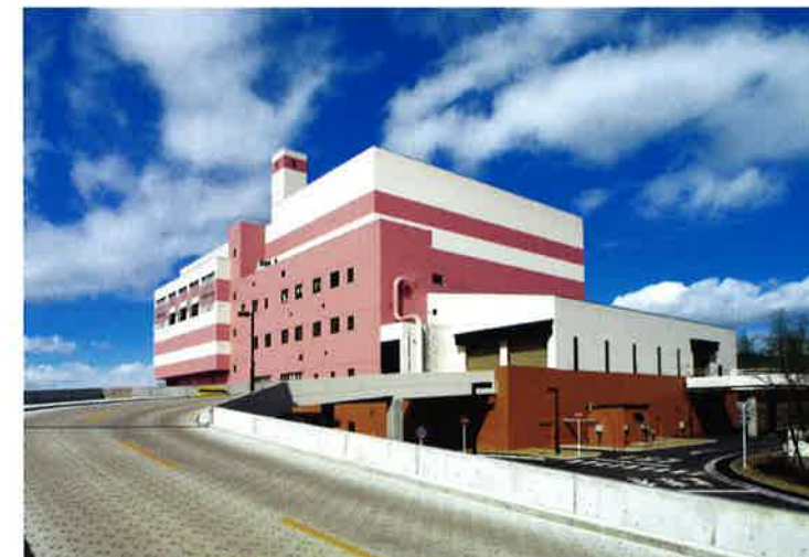
Clean center, Morioka-Shiwa Environmental facility union 80 tons/day × 2 furnaces (JFE High-Temperature Gasifying and Direct Melting Furnace) . 1,990kW of power generation, completed in 2003.
