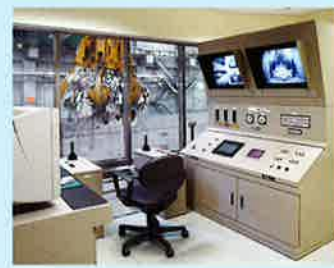
B Waste crane operation room
