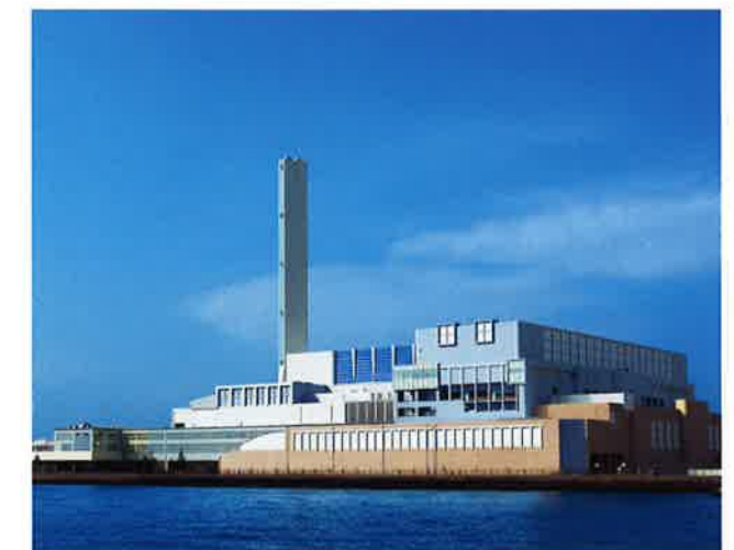
Kanazawa Refuse Incineration Plant. Yokohama 400 tons/day × 3 furnaces (JFE-VØLUND Grate). 35,000kW of power generation, with 60 tons/day Ash Melting Furnace (bottom ash), completed in 2001.
