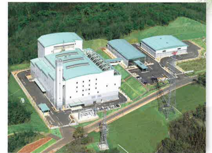
■ North Ishikawa RDF center <Completed March 2003> Fluidized bed type gasification melting furnace (Treatment volume: 80t/day x 2 furnaces, Power generated: 7,000kW)
