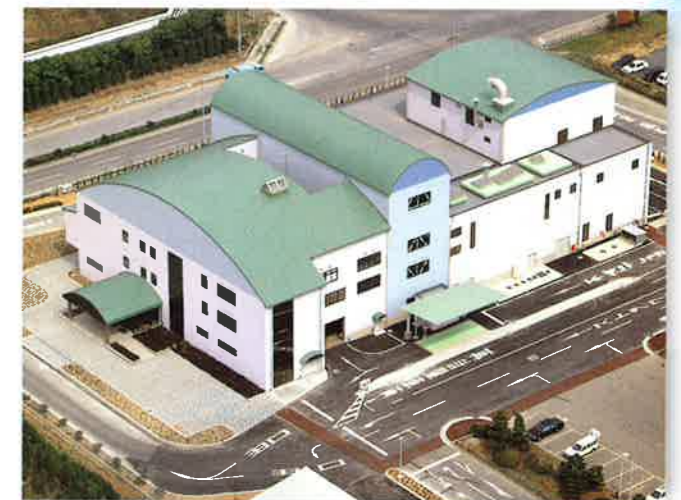
■ Ube Municipal Recycling Plaza <Completed March 1995> (Treatment volume: 70t/5h)
