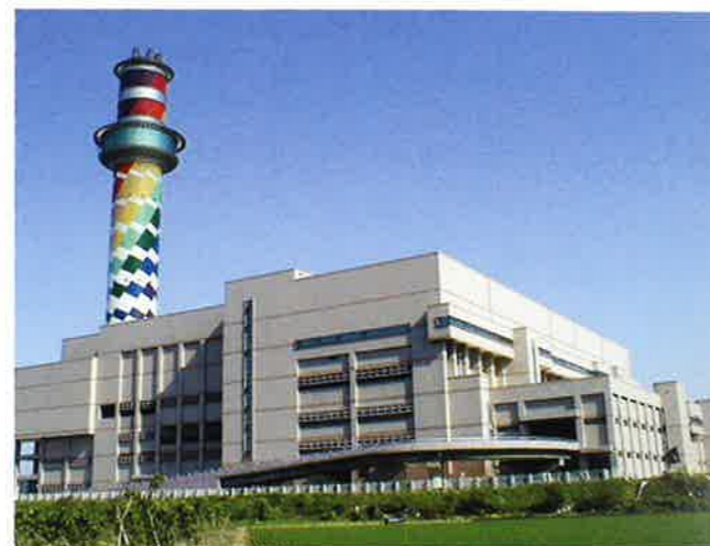
■ Taipei City, Government Environment Agency <Completed July 1998> Stoker type refuse incinerator (Treatment volume: 450t/day x 4 incinerators, Power generated: 48,000kW)
