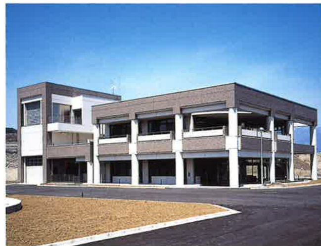
■ Asashina Purification Center <Completed March 1996> (Treatment capacity: 1,340m 3 /day x 2 systems)
