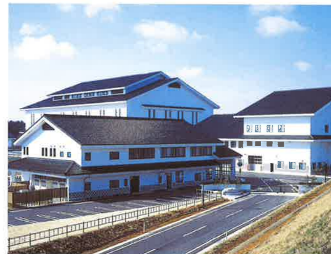
■ Okunoto Refuse Recycling Center, Refuse derived fuel manufacturing facility <Completed March 2003> (Treatment capacity: 24t/day x 2 systems)
