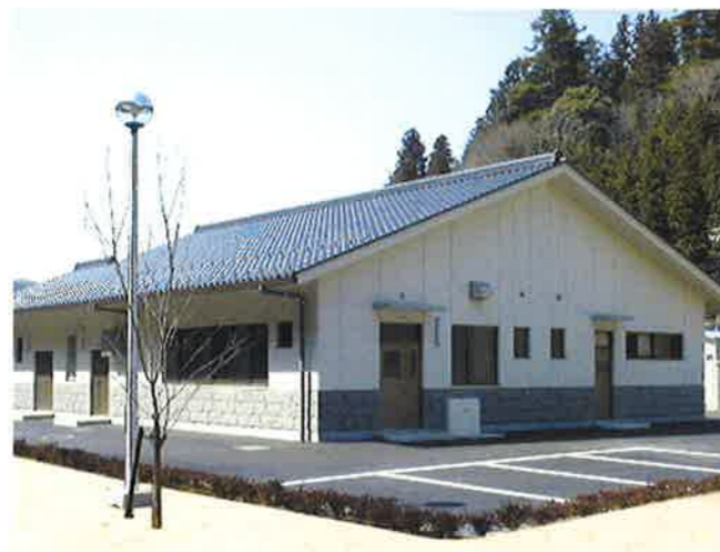
■ Hiroshima Prefecture, Jinseki County, Jinsekicho, Rural community sewerage Treatment facility <Completed March 2001> (Treatment capacity: 392m 3 /day)
