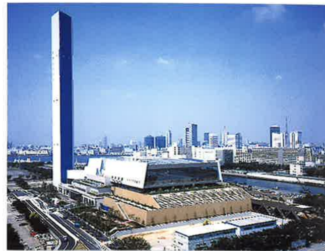
■ Citizen Association of TOKYO 23, Chuo Incineration Plant <Completed July 2001> Stoker type refuse incinerator (Treatment volume: 300t/day x 2 incinerators, Power generated: 15,000kW)
