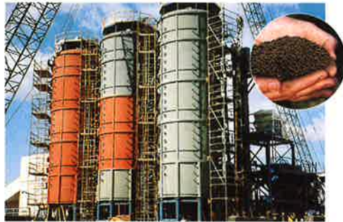
Hitz-Seghers sludge dryer-palletizer *12
