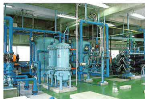
Sea water desalination system (Reverse osmosis process)*15
