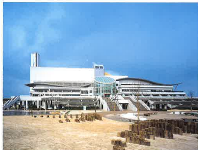
■ Fukuoka City, Clean Park Rinkai <Completed March 2001> Stoker type refuse incinerator (Treatment volume: 300t/day x 3 incinerators, Power generated: 25,000kW)
