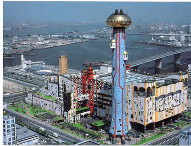
■ Osaka City, Maishima Plant <Completed April 2001> Stoker type refuse incinerator (Treatment volume: 450t/day x 2 incinerators, Power generated: 32,000kW)
