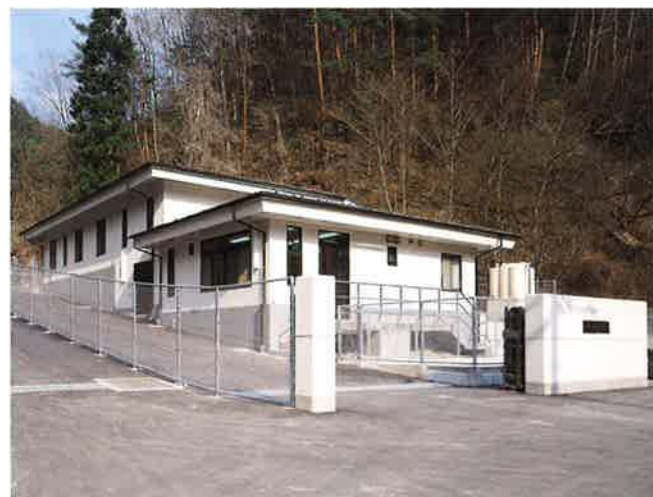
■ Matsukawacho General Waste Landfill Disposal Site <Completed March 2001> Leachate treatment system (Treatment capacity: 25m 3 /day)
