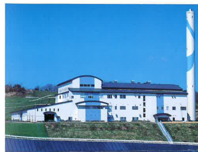
■ Niigata Prefecture, Environmental Protection Foundation (EcoPark Izumozaki) <Completed March 1999> Rotary kiln type incinerator (Treatment volume: 50t/day)
