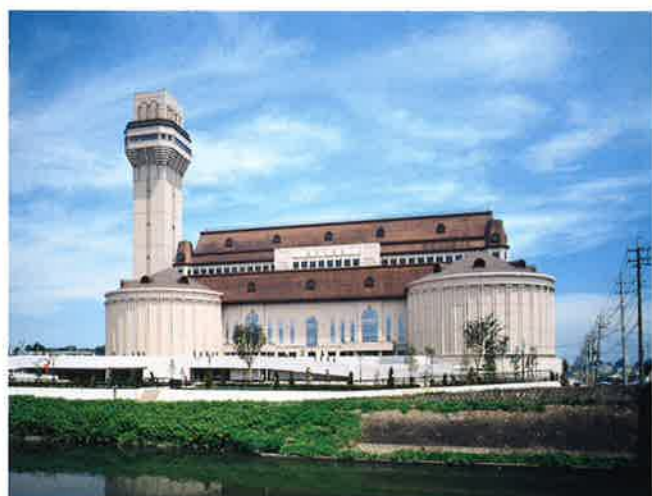
■ Resource and Environment United-Cities of Saitama East, Plant #1 <Completed September 1995> Stoker type refuse incinerator (Treatment volume: 200t/day x 4 incinerators, Power generated: 12,000kW x 2 facilities)
