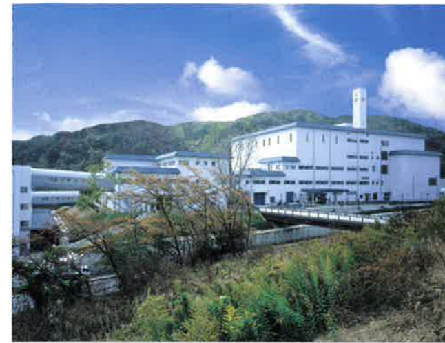
■ Sakurai City Clean Park <Completed November 2002> Fluidized bed type gasification melting furnace (Treatment volume: 75t/day x 2 furnaces, Power generated: 1,990kW)
