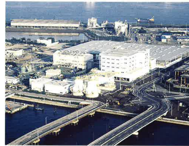
■ Citizen Association of TOKYO 23, Chubo nonflammable refuse treatment center <Completed September 1996> (Treatment volume: 900t/19h x 2 systems)
