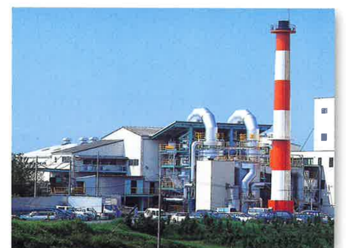
■ Company N (medical waste treatment center) <Completed July 2000> Vertical incinerator (Treatment volume: 14t/8h x 2 incinerators)
