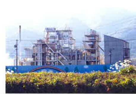
Fluidized bed type gasification melting furnace*3
