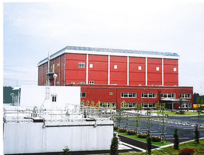
■ Ichibanya Co. Ltd., Tochigi Plant, Food product manufacturing waste water treatment facility <Completed September 1999> (Treatment capacity: 300m 3 /day)
