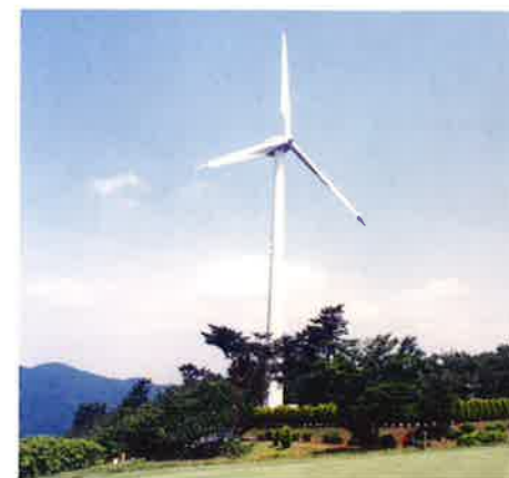
Wind power generation system*17
