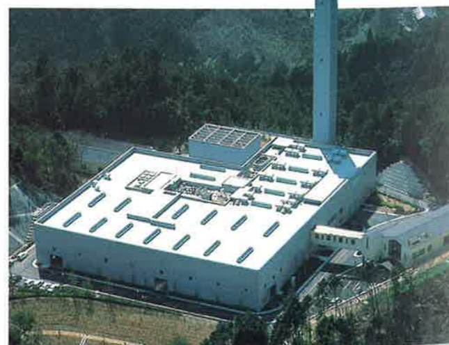
■ Minami-Kawachi Incineration Facility Union, #2 Incineration Plant <Completed March 2000> Stoker type refuse incinerator (Treatment volume: 95t/day x 2 incinerators) Burner type ash melting furnace (Treatment volume: 38t/day x 1 furnace)
