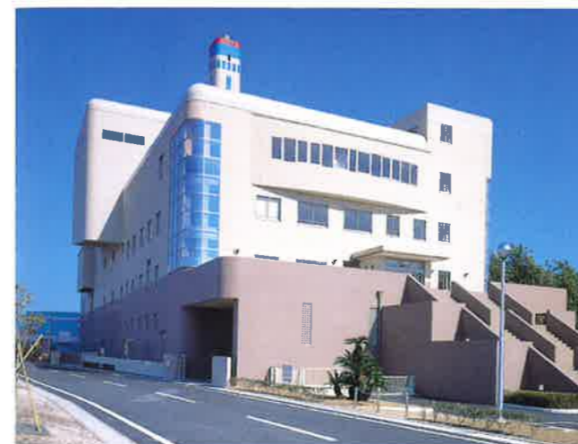
■ Yoshidacho-Haibaracho Regional Facility Union, San-R <Completed March 1999> Fluidized bed furnace (Treatment volume: 33.5t/day x 2 furnaces)
