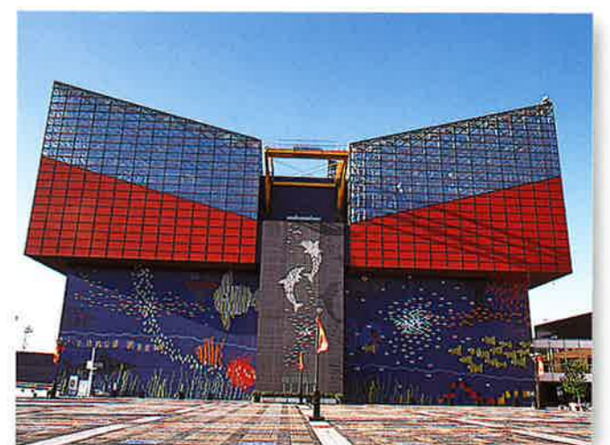
■ Osaka Tempozan Aquarium "Kaiyukan", Aquarium water treatment facility <Completed August 1990> (Total water volume in aquarium: 11,000m 3 )
