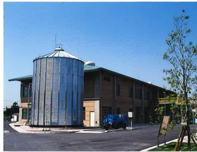
■ Nara Municipal Water Purification Center, Sludge reconditioning and treatment facility <Completed March 2003> (Treatment volume: Human waste 31kL/day, Purification tank sludge 59kL/day, Organic kitchen waste: 3.4t/day)
